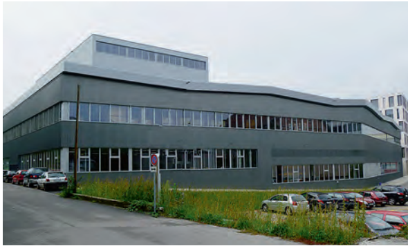
Brugg Kabel AG, H14, Brugg, Switzerland
